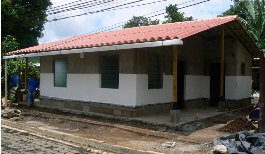
Figure 2: Prototype cane and mortar house, completed in 2012 (El Salvador Project, 2012). © Sebastian Kaminski
